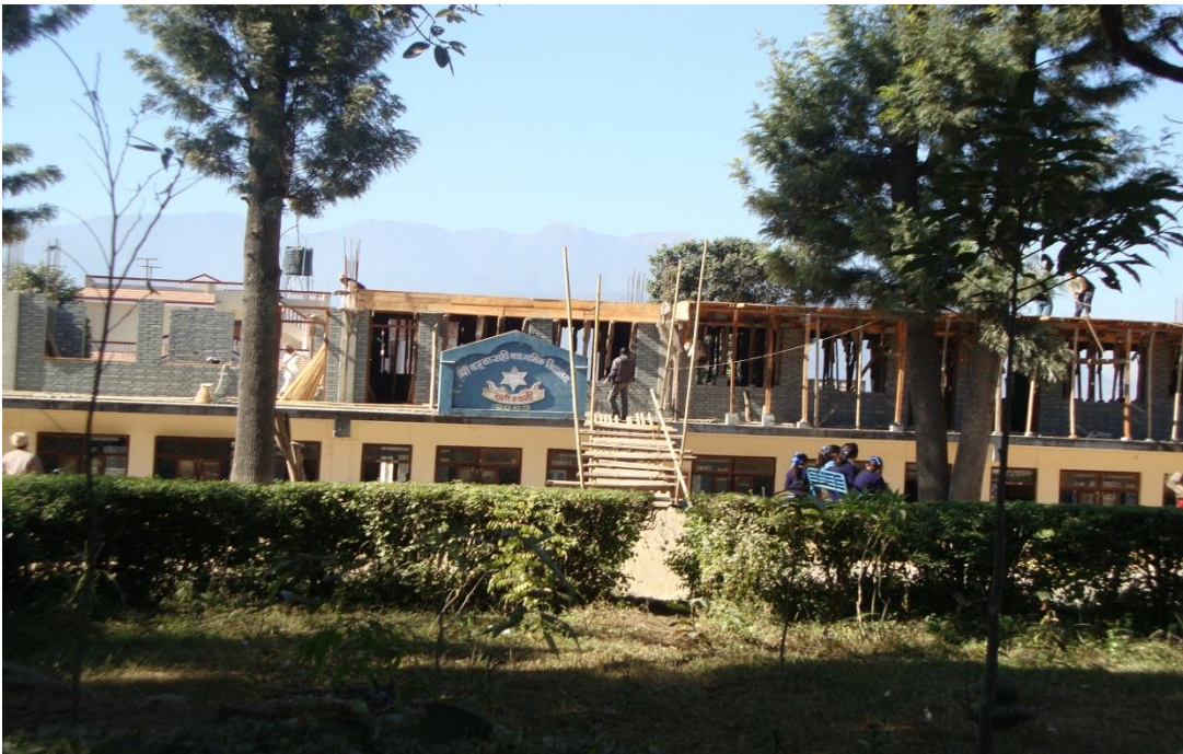
Ongoing construction of Bajrabarahi Higher Secondary School
